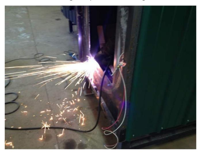
This leaves the stove's water jacket plate only up to the firebox. All cracks are repaired and the water jacket is pressure tested for leaks. This insures the stove will be in good working order when complete.
